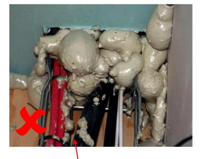
Forward planning of your fire protection requirements will mean choosing the correct method at the point of construction and prevent retrofitting of potentially unsuitable materials. Its easier to work with products like ablative coated batts at the point of first fix rather than trying to retrofit a solution that potentially wont meet the manufacturers install standards.
