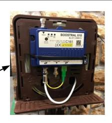
**External Termination Box (ETB)** Coax cables from Internal locations coiled with a 150mm tail. The ETB in Fibre areas is larger than our usual model, please bear this in mind when positioning the entry point to your property. We recommend access to the side of the property rather than the front. The ETB measures 250x250x120.
