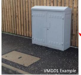
**Choosing a Cabinet Location** - Cabinets are best sited against property gable ends or against retaining or boundary walls where they are both protected from vehicle damage and as un-obtrusive as visibly possible to your site.
